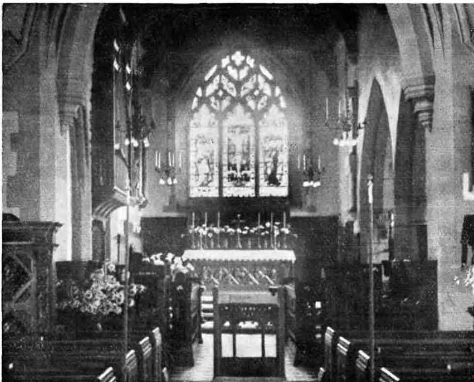
HARTHILL CHURCH INTERIOR showing Chancel restored in 1895 A.D.
